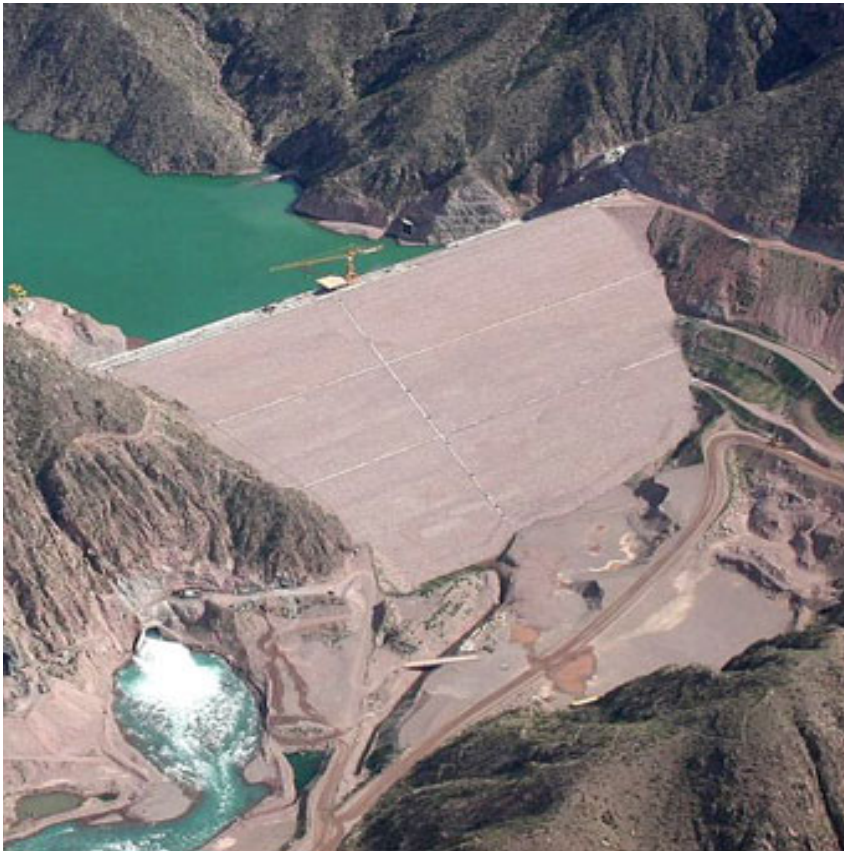
Potreriillos Dam Argentina
